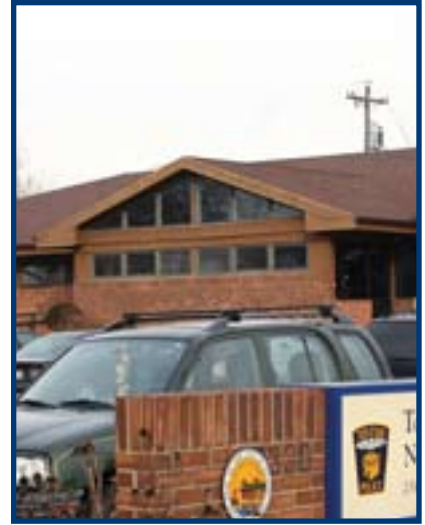
Northwest District Station 2330 West Sylvania Avenue
