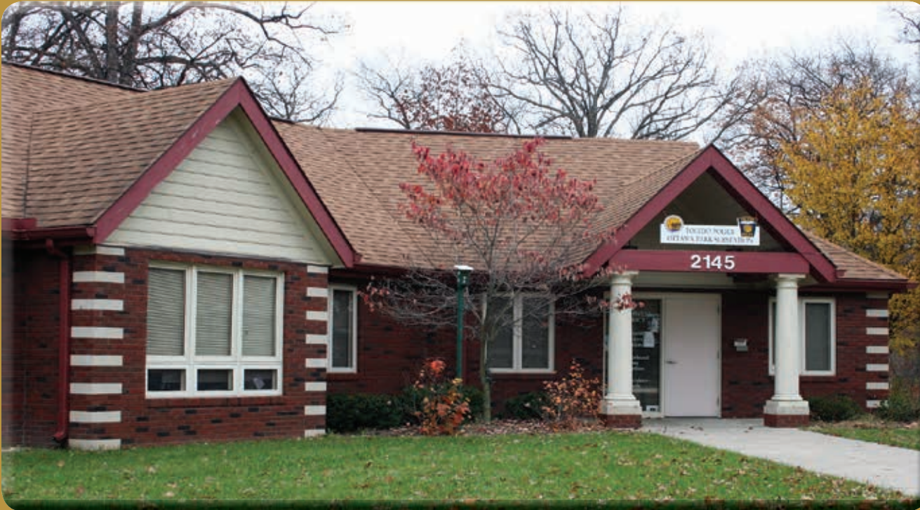
Ottawa Park Substation 2145 N. Cove Boulevard
