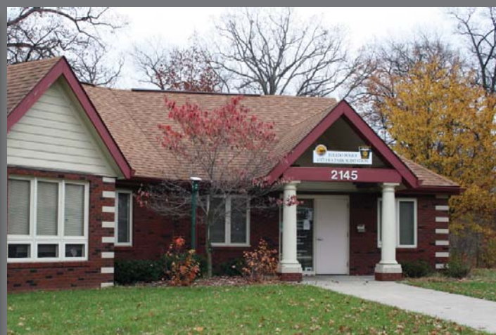
Ottawa Park Substation 2145 N. Cove Boulevard Toledo, OH 43606 419-936-3852
