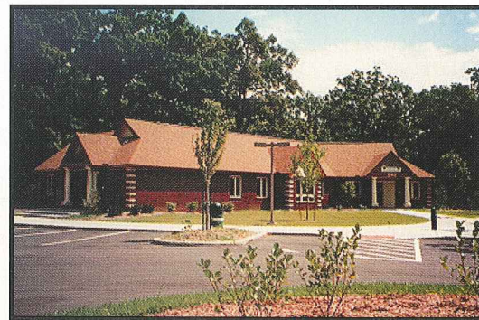
Ottawa Park Substation
