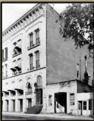
Superior Street Police Station
