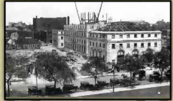
The Safety Building nearing completion.
