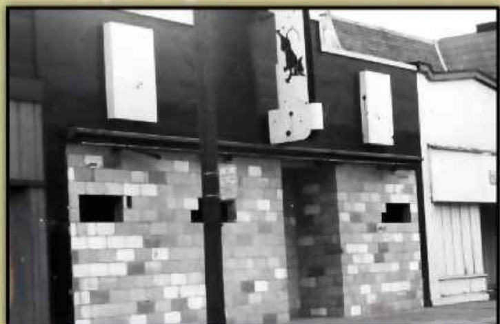
The Black Panther Headquarters, in the 1300 block of Dorr Street, was located in the former Sepia Theater. The building has since been razed.
