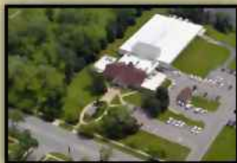
An aerial view of the Toledo Police Range (the large white building to the rear of the station) at Scott Park.
