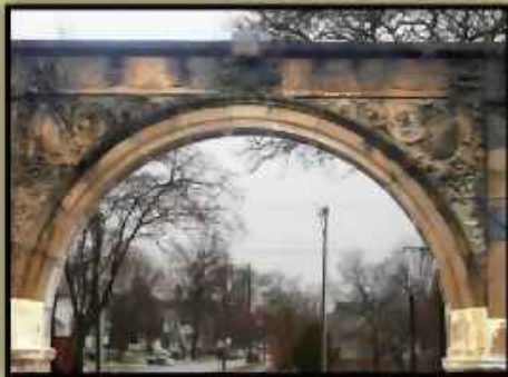
The Jackson Street arch as it stands today in the park at 222 Main Street on the East Side.
