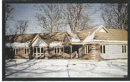
Ottawa Park Substation 2145 N. Cove Boulevard
