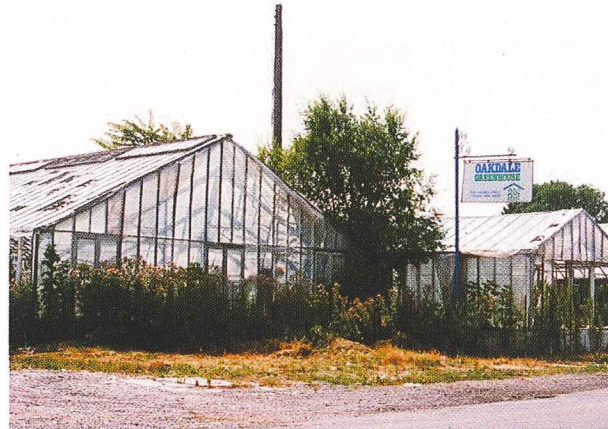
The former Oakdale Greenhouse, before demolition
